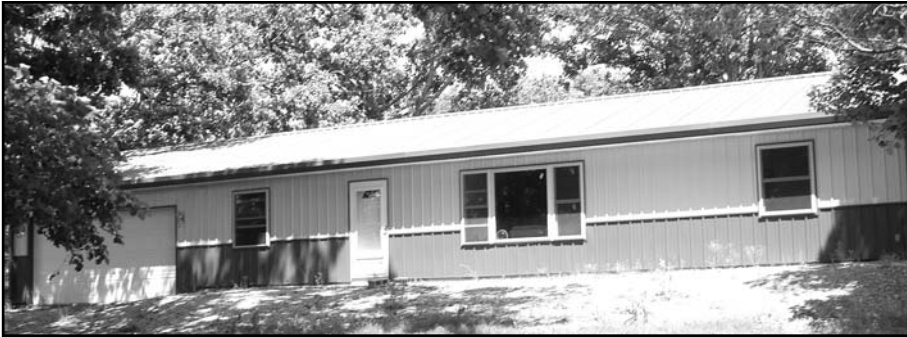
Above is an all-steel house in Mountain Home built by Cook's Metal Building Supply, who provided the concrete work, framing, and exterior steel siding and roof.
