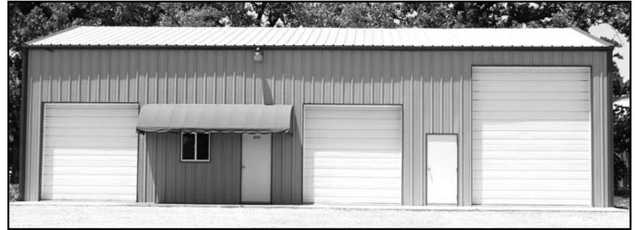
Above is an all-steel commercial building, located on Hwy 5 S in Mountain Home built by Cook's, who provided the concrete work, framing, and exterior steel siding and roof.
