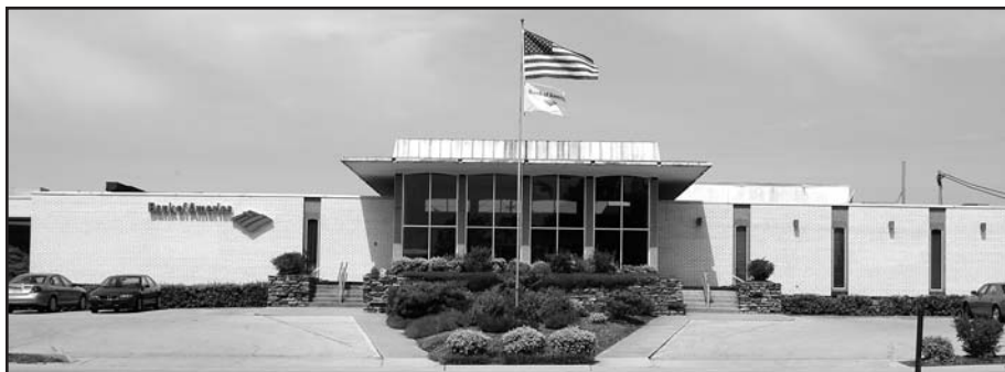
650 South Street - Mountain Home - 870-425-5171
